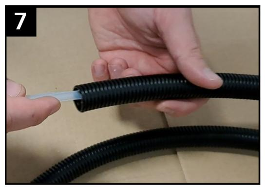
To prepare the pressure sensing hoses, feed the two hoses through the conduit.
